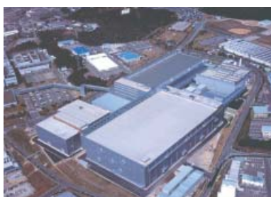
SCE semiconductor fabrication facilities
